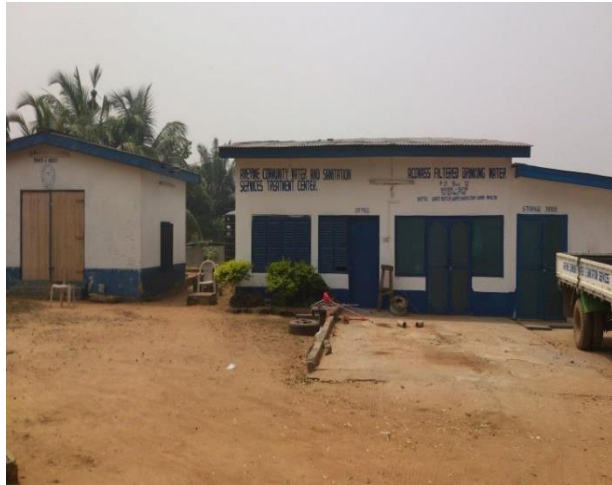
Aveyime Water Treatment Centre
